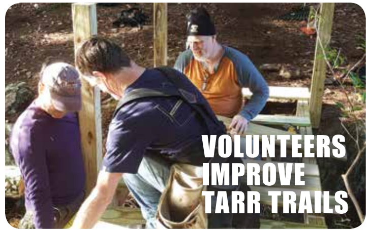
Volunteers building bridge on Tarr Sanctuary trail.
